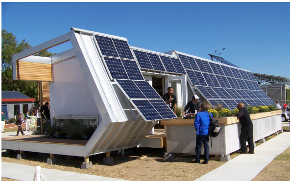
Figure 5. South and west elevations, Project Solar House. Note the form has been canted to maximize solar production. Source: (Gabbard 2007).
