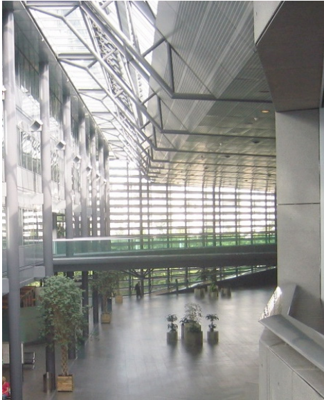
Figure 4: Grenoble Courthouse, 1994-2002. Breathable facade. Single-glazed outer skin, 40 mm (1.5 in) wide air space, double-glazed IGU inner skin. Source: (Author)
