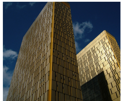
Figure 9: European Court of Justice, 2007. Kirchberg, Luxembourg. Breathable facade. Architectural metal elements within 150 mm (6 in) wide air space. Source: (CC-BY-SA: sprklg)
