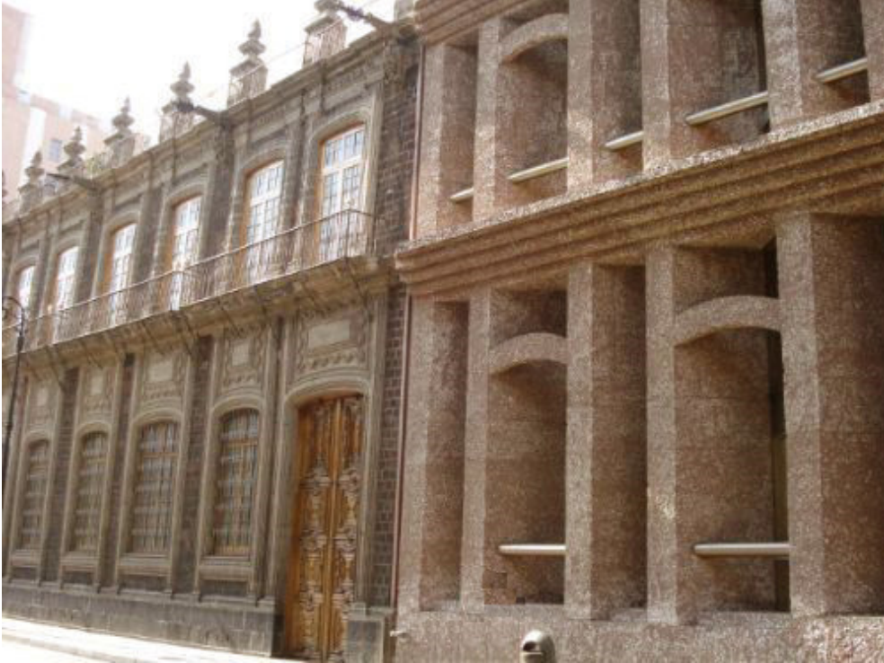
Figure 1: Banamex Central Headquarters, Mexico City by Teodoro Gonzalez de Leon and Abraham Zabludovsky
