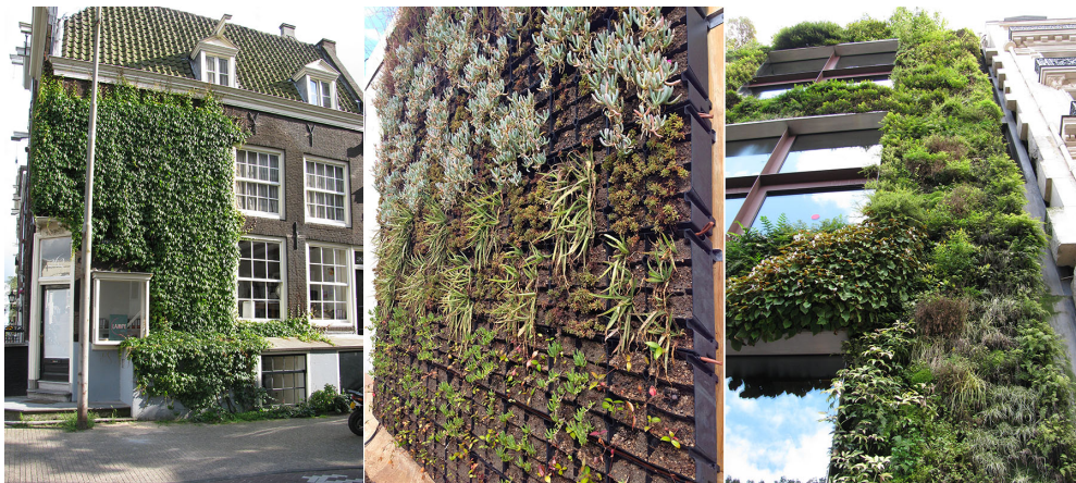
Figure 1. Green wall systems include vines with adhesive root systems grown directly on walls (left image) modular PVC-based systems (middle) and hydroponic systems constructed from fabrics (right). Source: Authors
