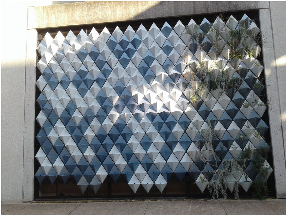
Figure 3: Southwest facing wall with 300 modules installed. Photo taken during the early morning. Source: Authors
