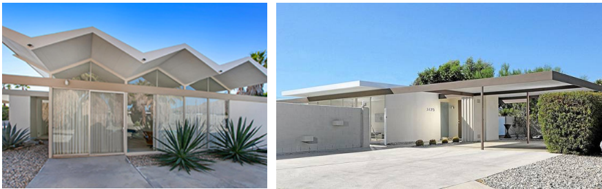
Figure 1: Prefabricated Steel Erection and Construction, Steel Houses, Donald Wexler, 1962
