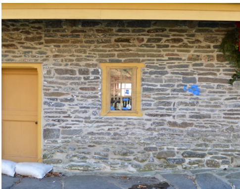
Figure 6. N.wall at thermocouples, RittenhouseTown
