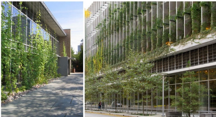
Figure 1: Examples of VGS on building facades (Left: Pritzker children's zoo at Lincoln Park Zoo in Chicago Illinois, Right: Rush Medical Centre in Chicago Illinois) ("Vines72.jpg (324×432)" n.d.) ("TL_Mar-2008_Rush.jpg (1200×900)" n.d.).
