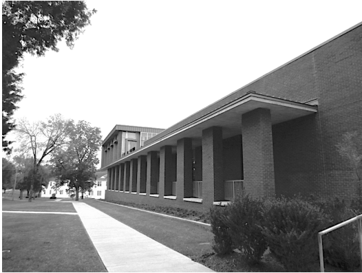
Fig 3 Thompson Center porch as shading device.
