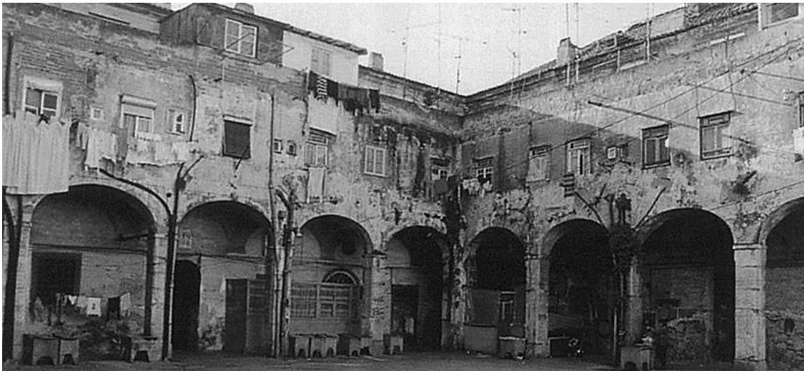
Figure 4: Courtyard of the Bernardas Convent transformed into lower class residences (Almeida, 2000)
