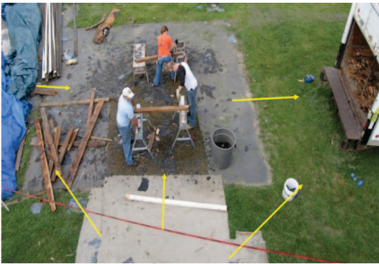
Photo 1: “Work triangle” for materials coming building under deconstruction
