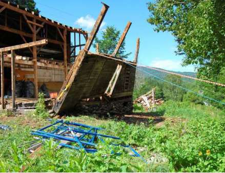
Photo 4: Back wall being removed by group effort
