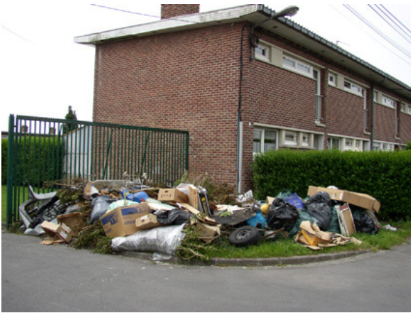
Figure 8: Entrance of a collective backyard. Source: (BazarUrbain 2005)
