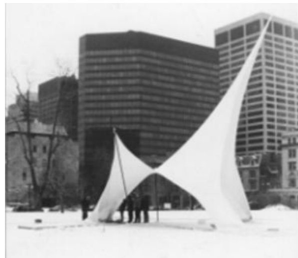
Figure 3: Nylon-reinforced, double-curved ice structure with free edges
