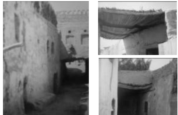
Figure 10: Rooms extends over a street below created the sabat, covered streets at Al-Qasr Village.
